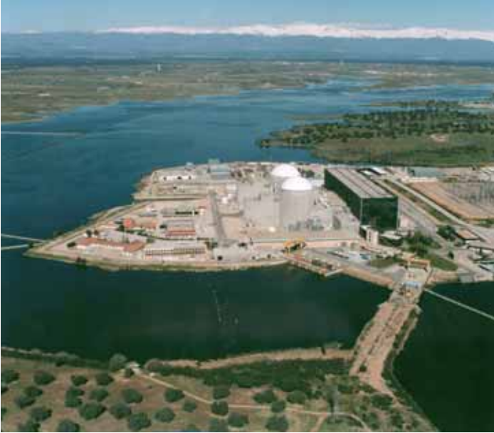
Located in Extremadura, not far from the border with Portugal, the Almaraz nuclear power plant was commissioned in the early eighties. It is the first Spanish plant that was equipped with Generation II reactors.
