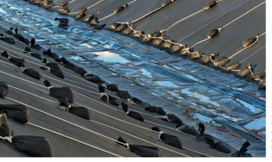
When one cell of this near-surface, very low-level waste repository operated by Andra (France) is full, it is covered with soil and revegetated.
