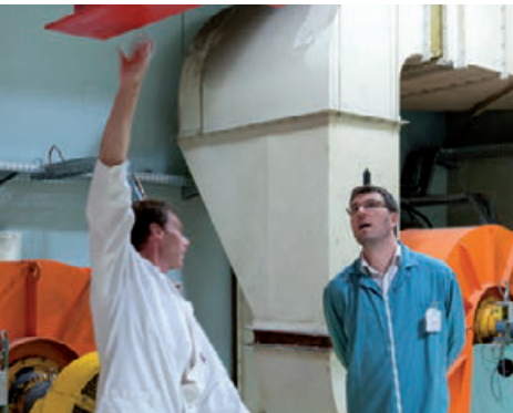
In-situ inspection carried out at the Institut Laue-Langevin's nuclear research facility in Grenoble (France) as part of the European stress tests.
