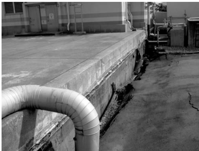
Subsidence of refilled soil after the 2007 tremor at Kashiwazaki-Kariwa NPP (western Japan).
