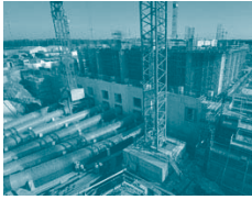
Construction work at Olkiluoto 3 NPP
