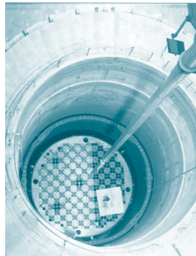
View into the open reactor pressure vessel on the reactor core during maintenance
