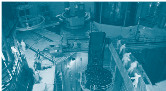
Scheduled shutdown at Lingao NPP (China)
