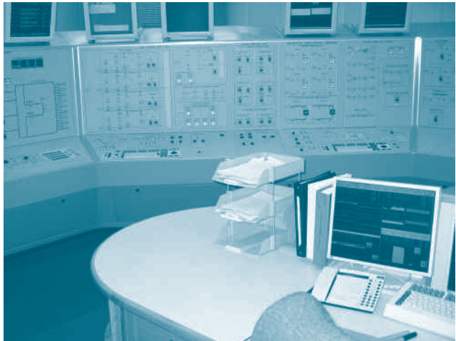
View of Control Room Training Simulator
