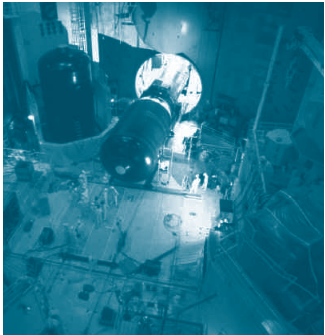
Steam generator replacement
