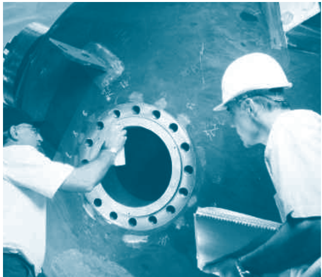
Visual inspection of a steam generator by the manufacturer
