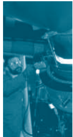
Maintenance work performed on a steam generator
