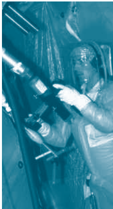
Maintenance work on steam generator tubes
