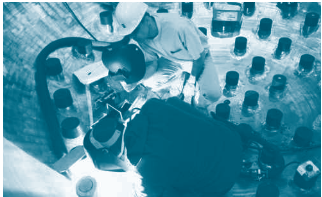
Visual inspection of a steam generator
