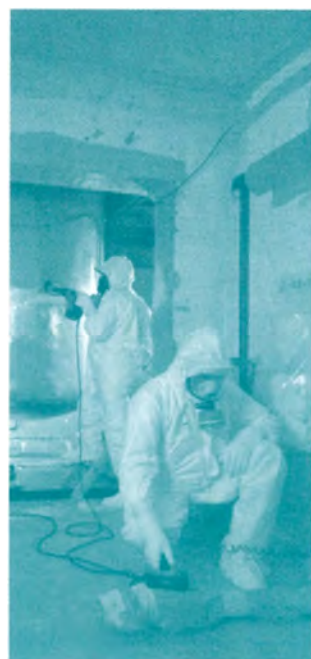
Dismantling of washer and piping.
