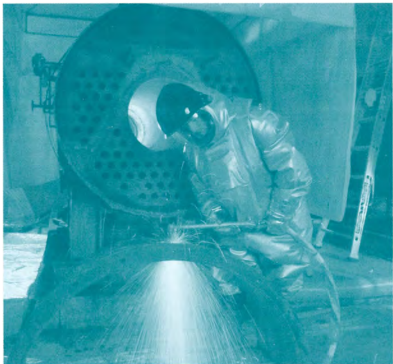
Boiler cutting performed using fire protection clothing.
