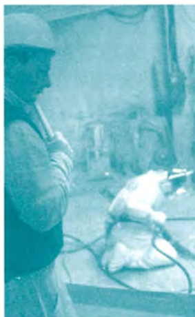
Decontamination of activated concrete parts.
