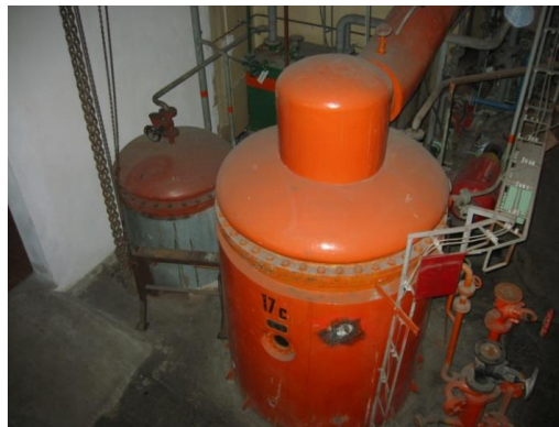
Fig.: Heater and Olde evaporator before dismantling
