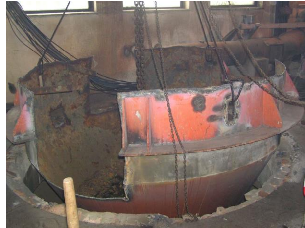
Fig.: The storage tanks before fragmentation and removal the bottom of tank
