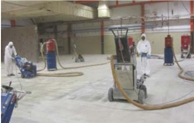
Decontamination of the floor
