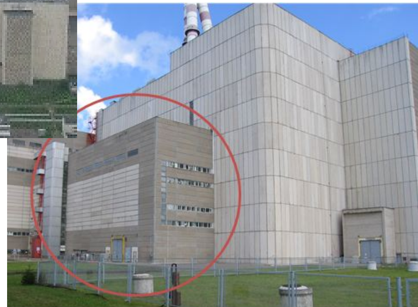
Building V1 of Ignalina NPP
