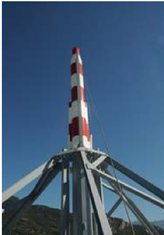
Release chimney of CDS
