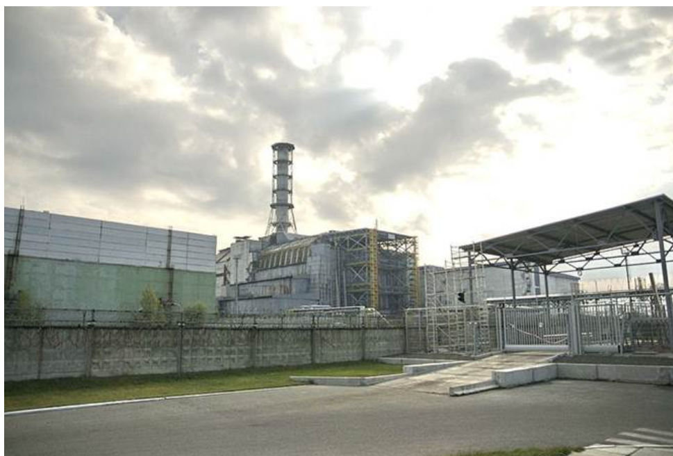
Fig. 7. Part of the perimeter of Shelter protected area with transport entrance gates and physical protection equipment
