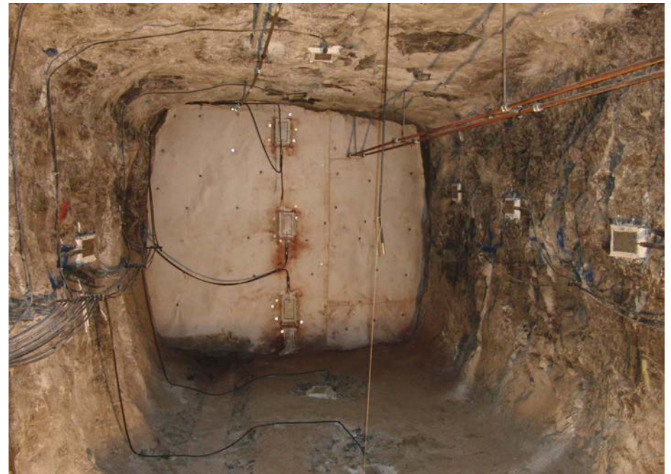
In situ-Test site before concreting (nearly full scale: length: 8 m)
