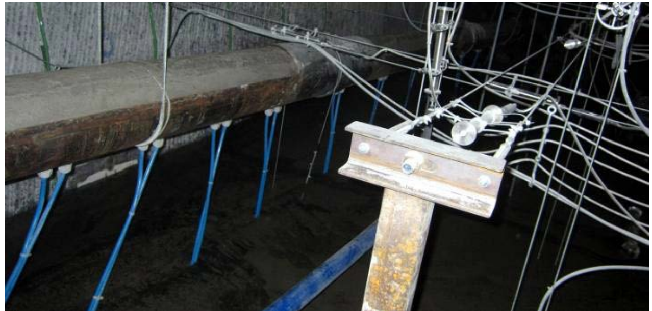
Concreting of the drift seal (484 m 3 - continous construction time: 20 h – 15. / 16. Dez. 2010)
