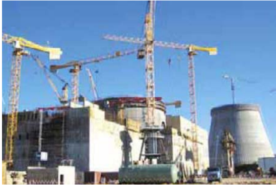
Novovoronezh NPP-II Unit 1 – 2014; unit 2 – 2015
