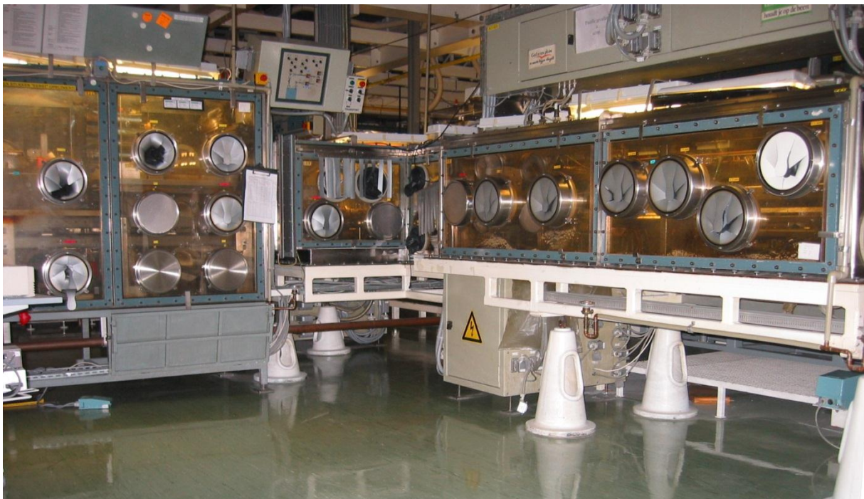
Fig. 1 : Glove boxes of the production line to be dismantled.
