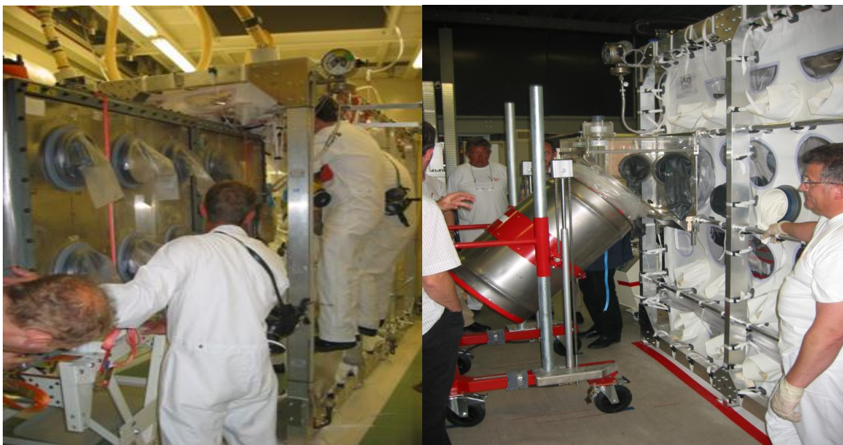
Fig. 2 : Left : glove box being inserted in frame for peditent. Right : peditent mounted around glove box, waste drum hooked up, ready for filling.
