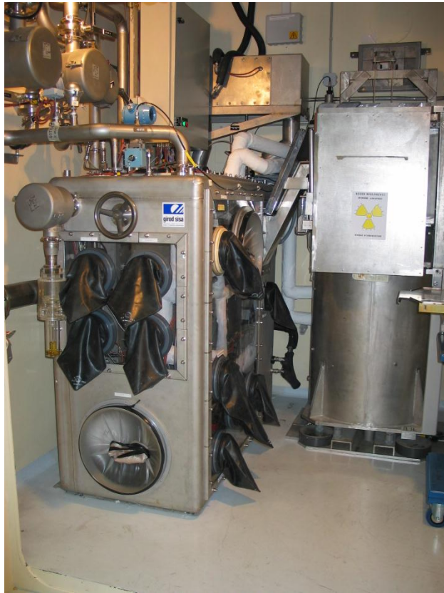
View of EPICUR facility
